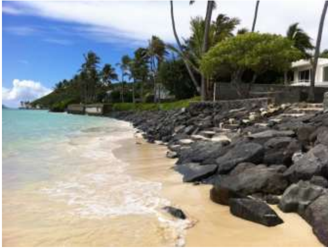
Beach loss fronting coastal armoring at Lanikai, Oahu.
