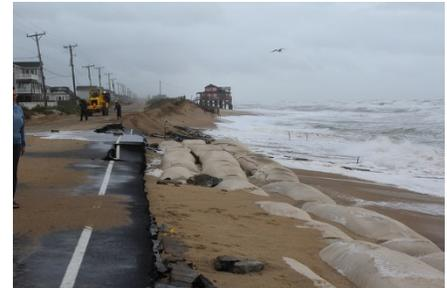
Erosion mitigation on NC 12 in Kitty Hawk, NC, Oct. 2015. Photo: County of Dare.
