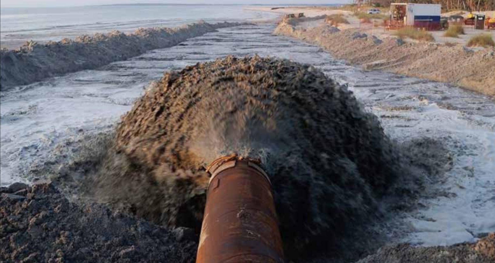
Figure 9. Overview of potential processes occurring during and after a sand deposition event during beach nourishment. (A, above) Deposition of anoxic/reduced sand. Compare with color of existing sand nearby (see Figure 7c) (Photo: N. Elko). (B, below) Potential processes following a sediment placement event. Arrows indicate fluxes of matter. See Figure 8 for more details on impacts.
