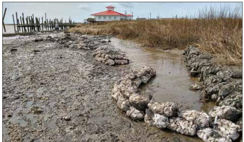
living shoreline treatments, an additional 700 shell bags were placed in cusps along the previous control areas, creating a total of 400 feet of contiguous living shoreline. This included a shell bag "wedge" at the most northerly end of the shoreline, where significant erosion was observed at the Bend control area.
